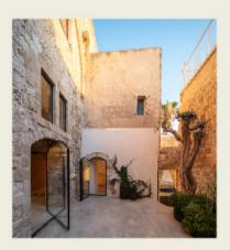
The original kurkar sandstone was intentionally uncovered, treated and exposed, while dark bronze frames and glass elements highlight the vaulted interior doorways, plastered ceilings and sea-views.
